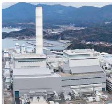
中国電力三隅発電所 The Chugoku Electric Power Co., Inc., Misumi Power Station
